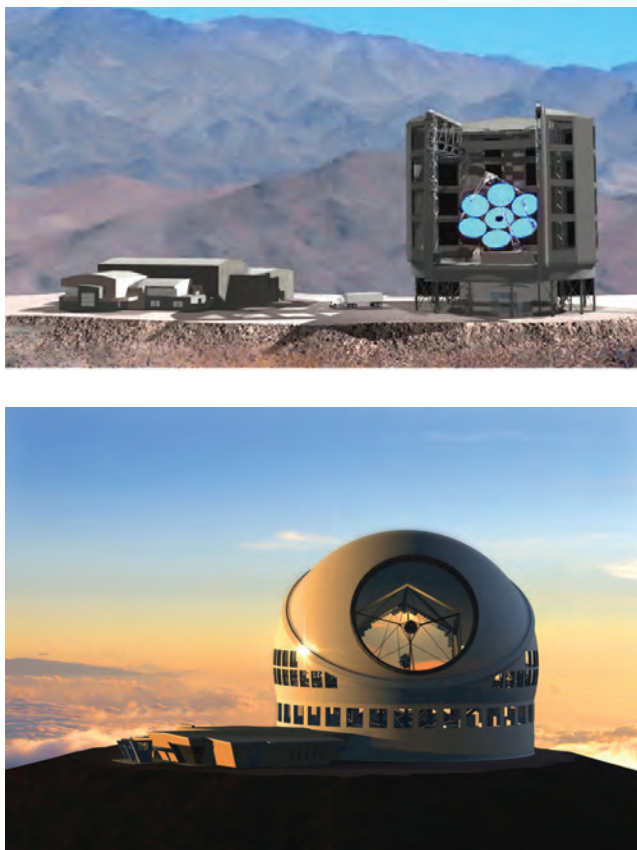
FIGURE 7.9 The two U.S. Giant Segmented Mirror Telescope projects. Upper: The Giant Magellan Telescope is a 25-meter-class telescope comprising seven 8.4-meter subapertures, one of which is already undergoing polishing. Laser tomography will provide adaptive optics correction in small fields over much of the sky, and correction for ground-level seeing will be incorporated over large fields. The baseline project includes an initial suite of three to four instruments to be selected in 2011 from eight concepts currently in development. Artist's rendering of GMT and support facilities at Las Campanas, Chile. SOURCE: Courtesy of GMT; image by Todd Mason/Mason Productions. Lower: The Thirty Meter Telescope primary mirror comprises 492 hexagonal segments with active control and a 30-meter-effective-diameter aperture. An on-axis segment has been cast and polished, and an off-axis segment is currently undergoing polishing. Nine instruments are planned for the first decade of operations, of which three are planned for first light. Most of these instruments operate in conjunction with sophisticated adaptive optics systems. SOURCE: TMT Observatory Corporation.
